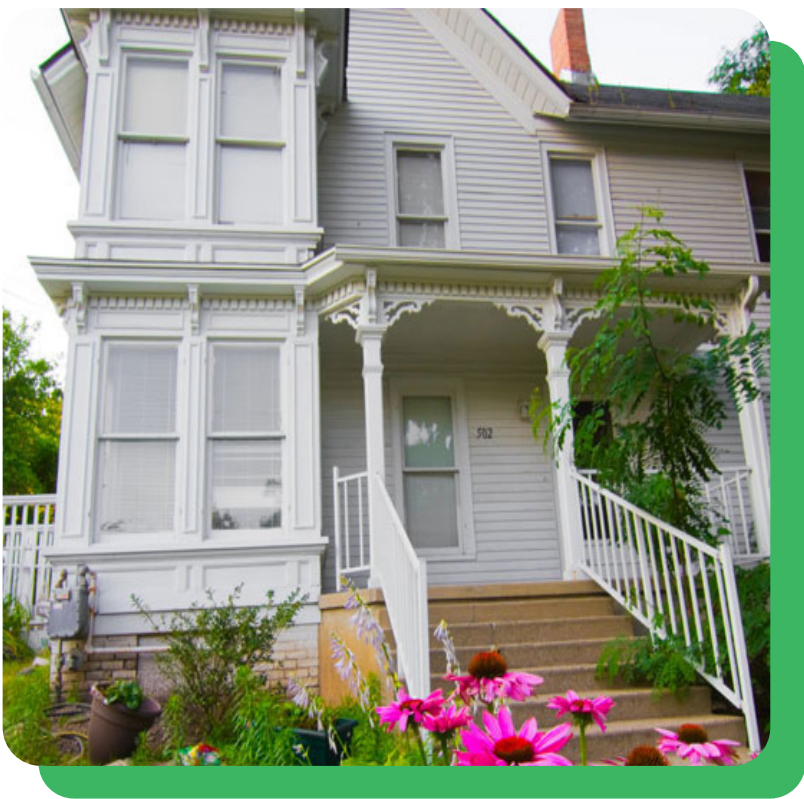
Spera Recovery Center 1
